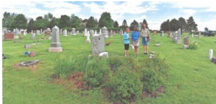
Barb Mallon, Joan Schoon and Dennis Mitchell inspect the progress of the project to clean and repair headstones at Bethlehem Lutheran Church Cemetery in Slater. RONNA FAARBOG/WJMS TRIBUNE
