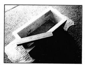
Note: <u>Do not oil</u> the foam sides. Cut the tape to remove the form pieces; they can be used again.
